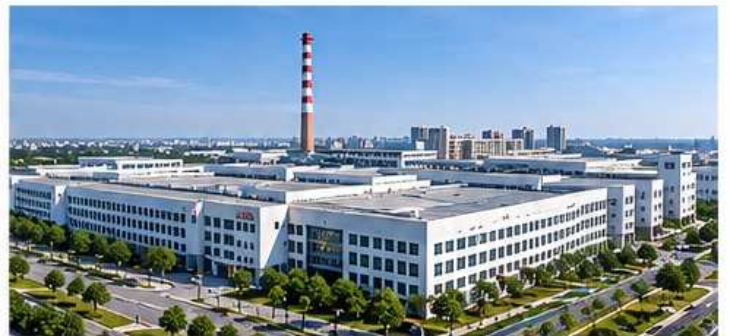
05 | Industrial Manufacturing Facility — Zhengzhou Industrial buildings
